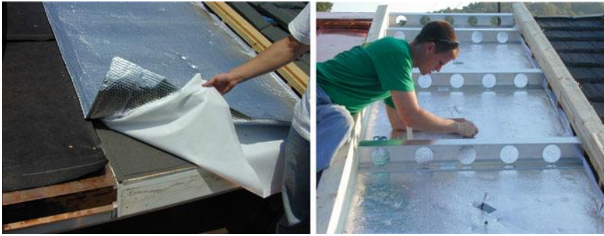
Figure 12: Roof assembly comprising of insulation and subverting air channels with two PCM insulation systems (Kośny et al. 2012)
